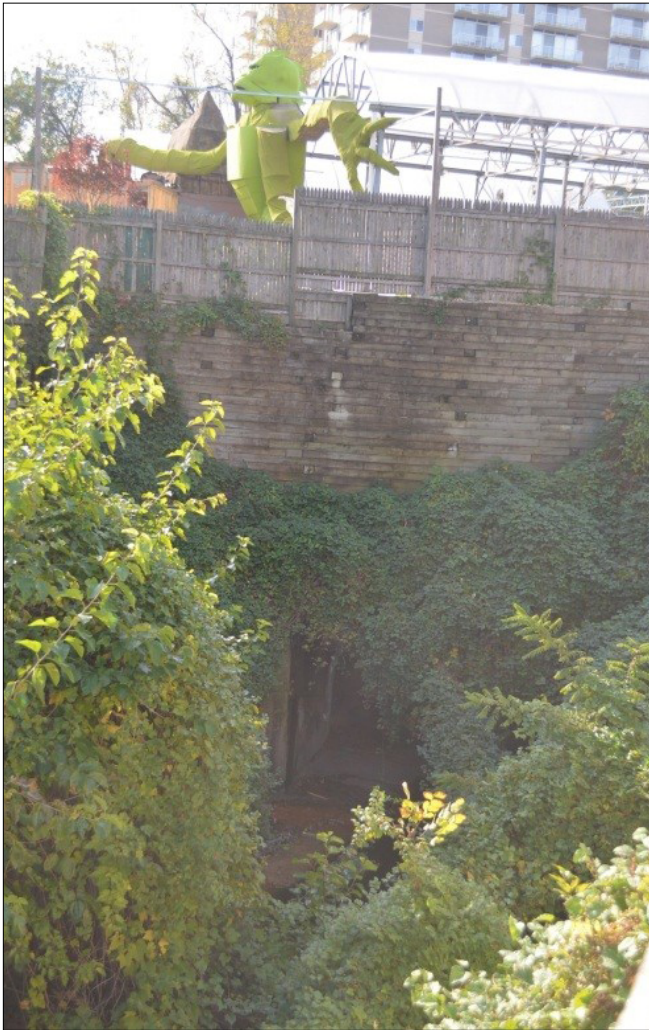
Entrance to American Plant Food's Willett Branch tunnel
