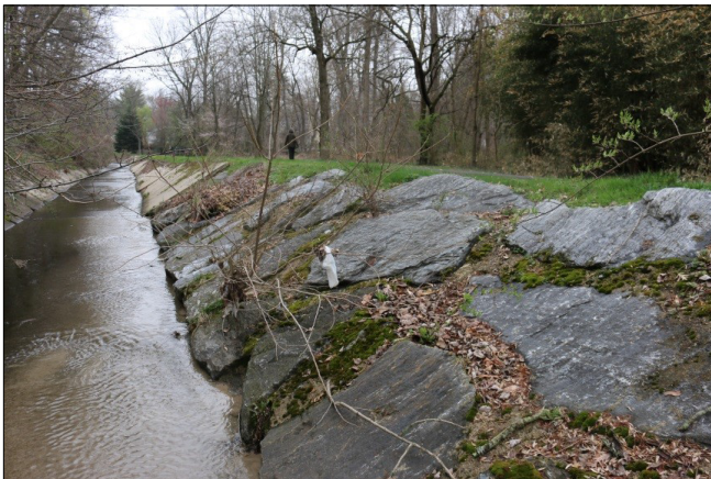
Figure C.8: Interim Stream Bank Repair without Concrete
