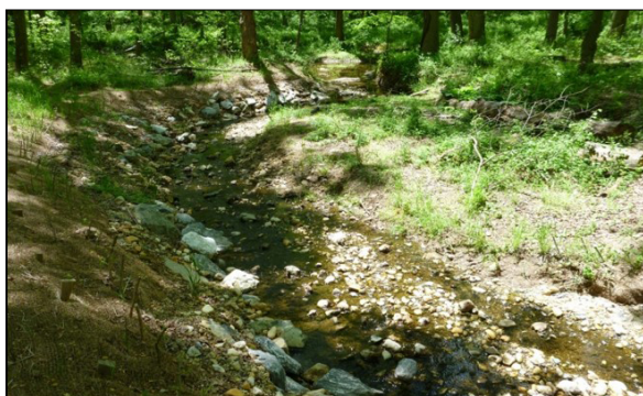
Restoration (Craddock St Tributary to Upper Paint Branch)
