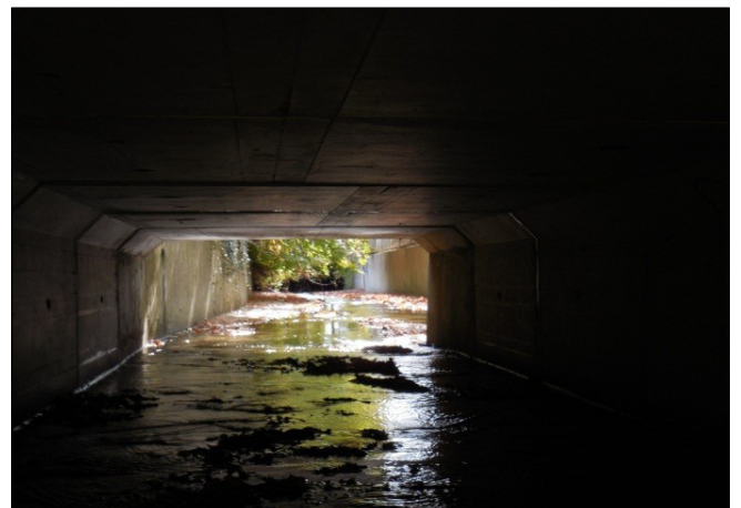
Inside the tunnel
